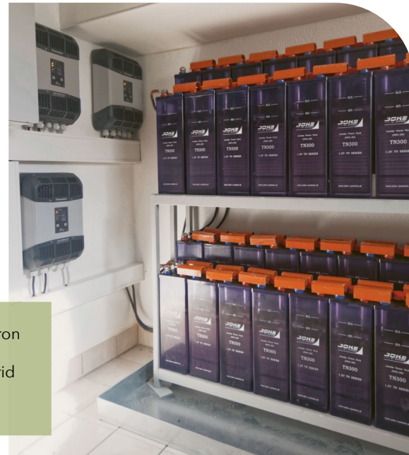
Installation with lead-acid batteries for backup and uninterrupted power supply in the Islamic University of Gaza in Palestine
