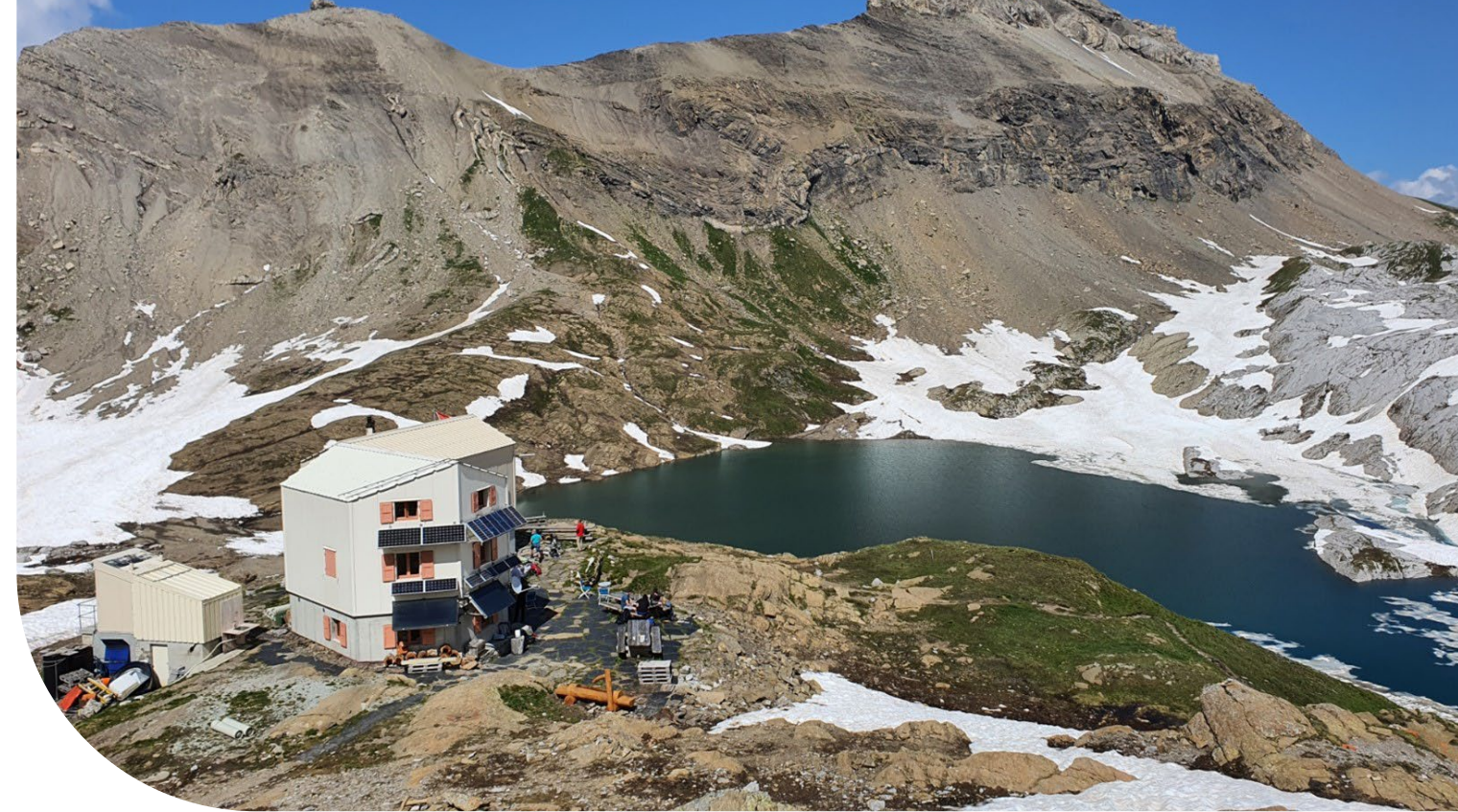
Cabane des Audannes: an appreciated trekking destination in the Alps, powered by solar and pico-hydro with a Studer system
