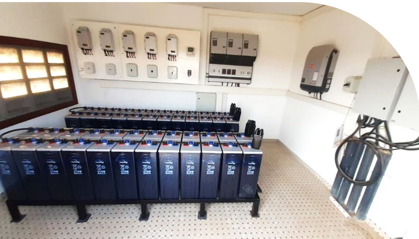
DC+AC-coupling system in South America
