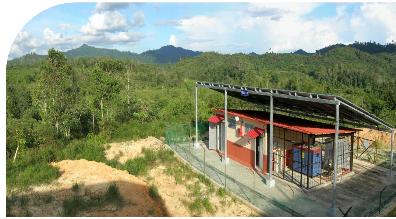
Hybrid systems for a school in Malaysia
