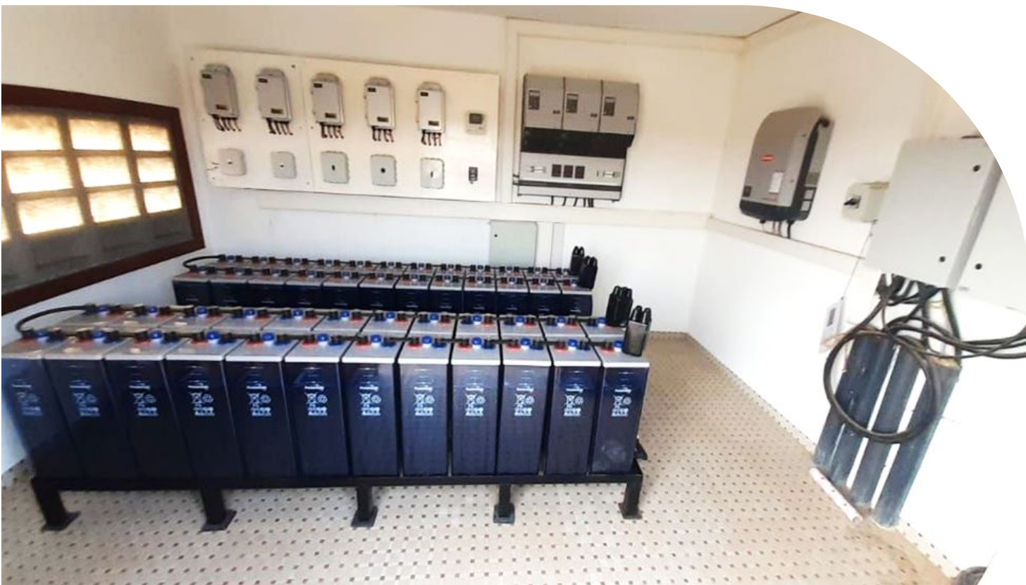
DC+AC-coupling system in South America
