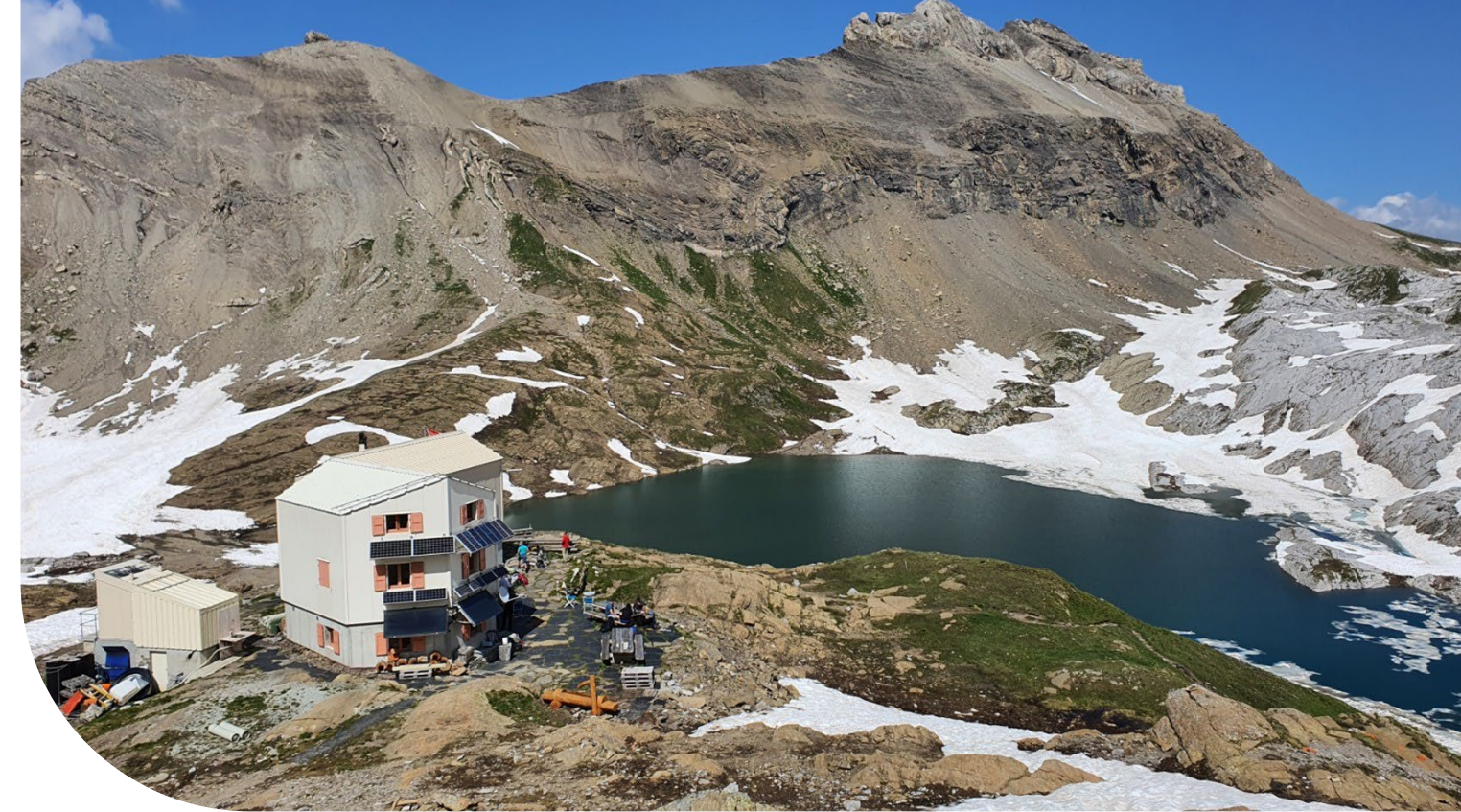
Cabane des Audannes: an appreciated trekking destination in the Alps, powered by solar and pico-hydro with a Studer system
