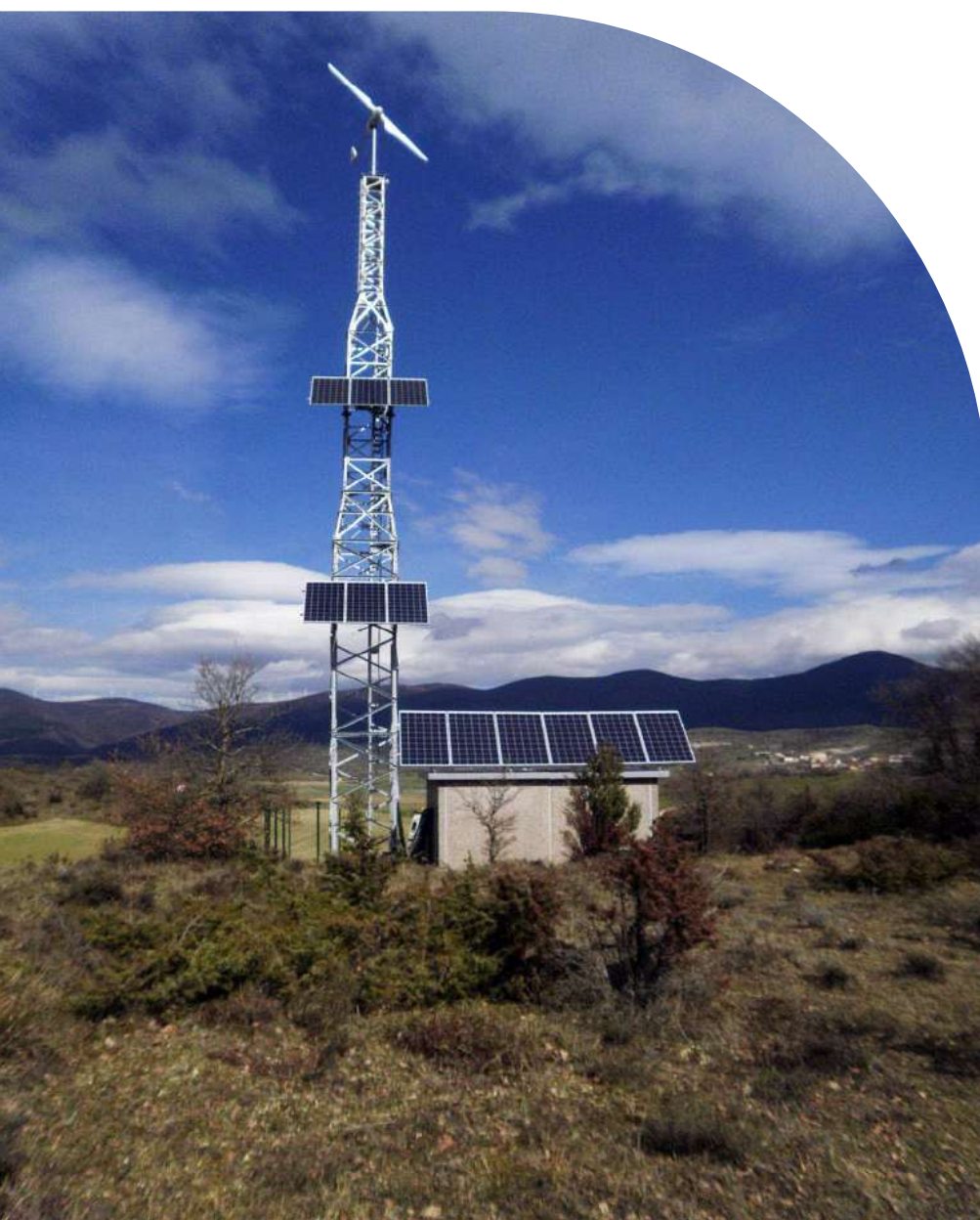
Itelazpi offgrid telecom tower, Spain
